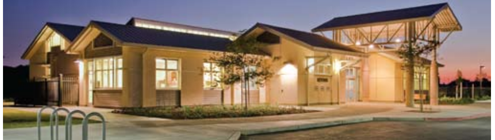
EXTERIOR AT TWILIGHT
