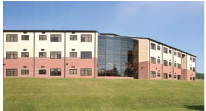
CLASSROOM WING EXTERIOR
