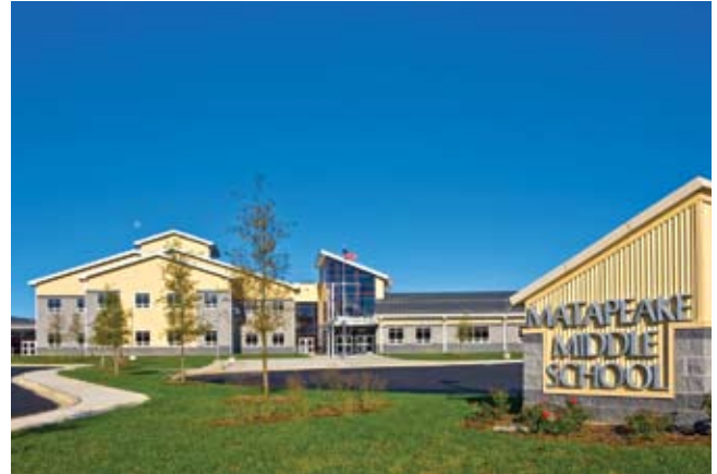
OVERALL FRONT ENTRANCE
