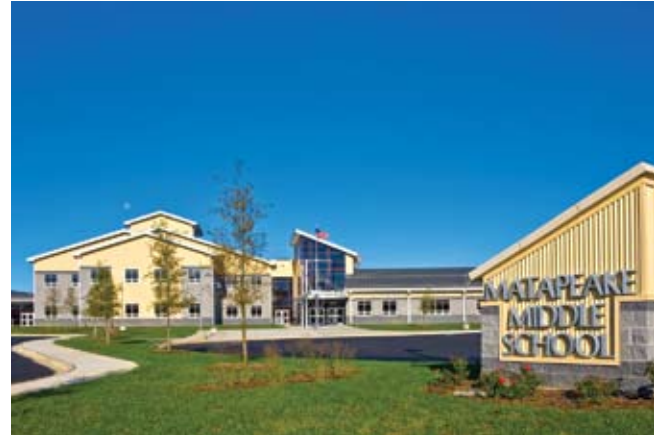
OVERALL FRONT ENTRANCE
