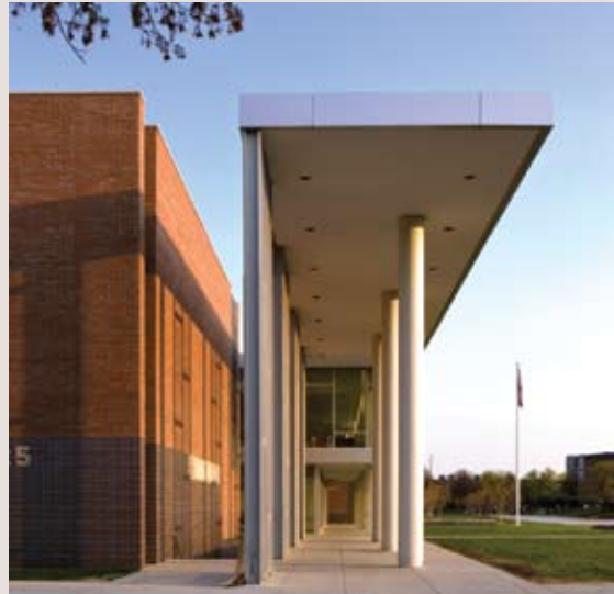
ENTRY CANOPY FROM 7TH STREET
