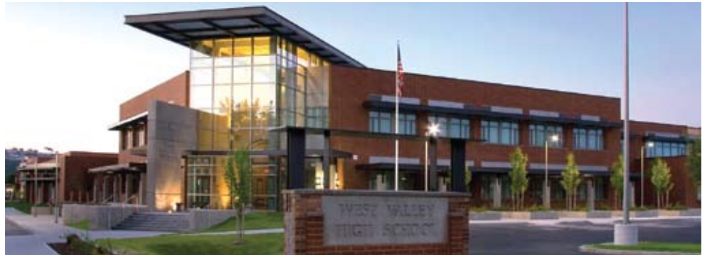
MAIN ENTRY AT SOUTHWEST CORNER
