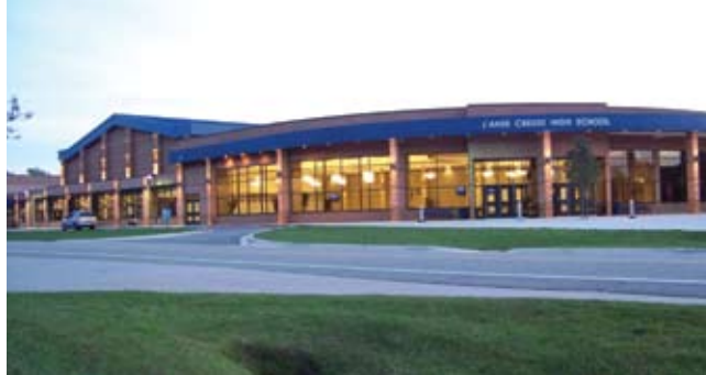
EXTERIOR OF ADDITION
