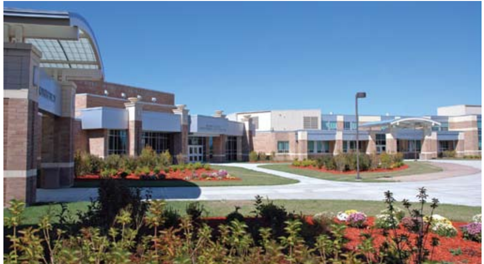
VIEW OF THE THREE PUBLIC ENTRANCES
