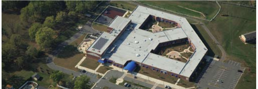
AERIAL PHOTO OF OVERALL BUILDING
