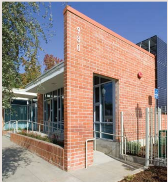
EXTERIOR WITH PHOTOVOLTAICS
