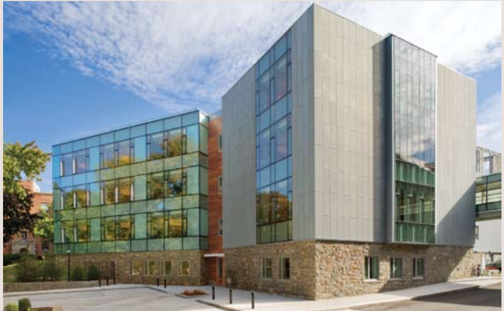
MIDDLE SCHOOL EXTERIOR
