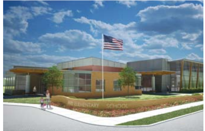
VIEW TOWARD BOTH ENTRIES FROM THE NORTHWEST
