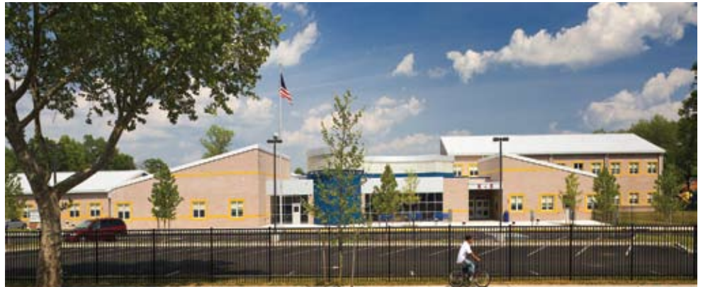
OVERALL FRONT EXTERIOR OF K-5 SCHOOL
