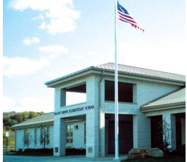
ENTRY LOOKING SOUTHEAST
