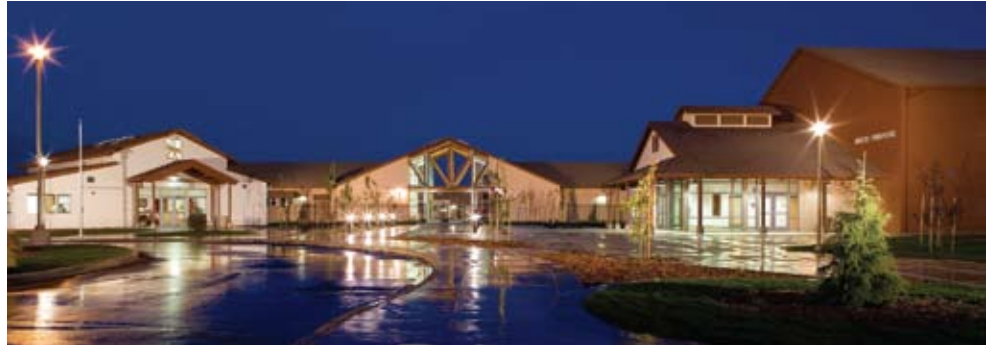
COMMUNITY CAMPUS ENTRY
