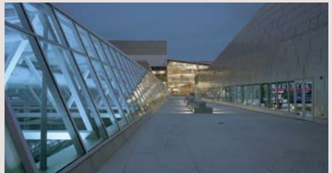
EXTERIOR PASSAGE BETWEEN NATATORIA
