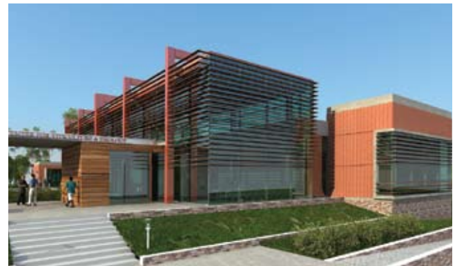
VIEW OF GRAND HALL FROM PARKING
