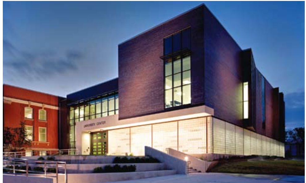
SOUTH ELEVATION AT TWILIGHT
