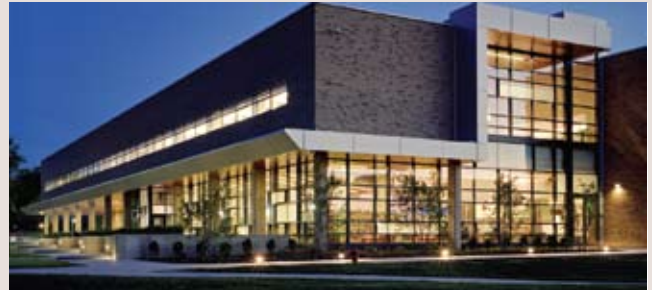
NORTH EXTENSION AT TWILIGHT
