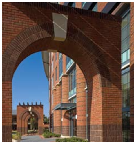
MALL ARCHES/LOOKING NORTH
