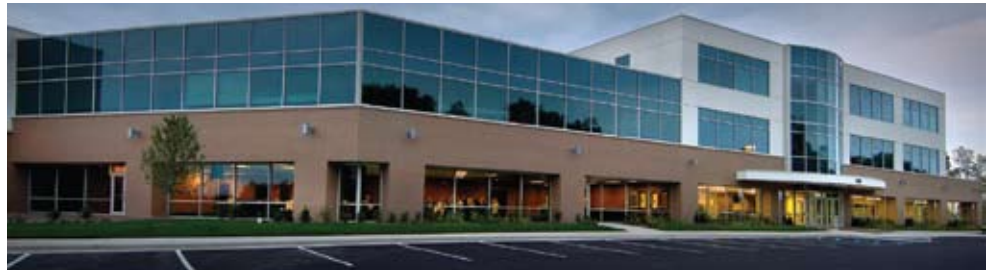
NORTH EXTERIOR FACADE
