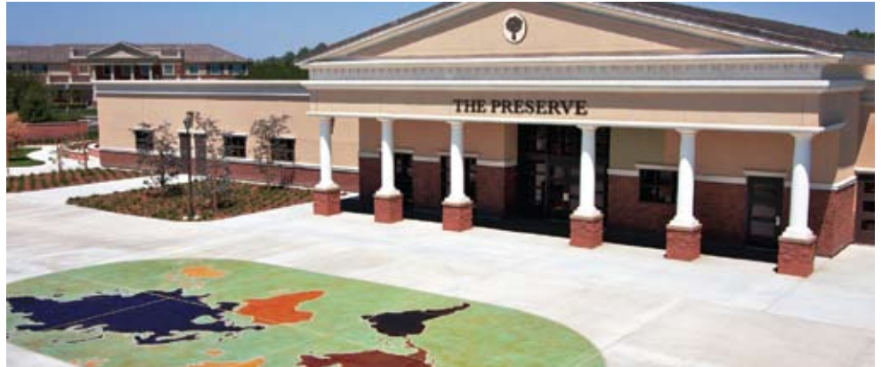
ADMINISTRATION AND ENTRY COURTYARD
