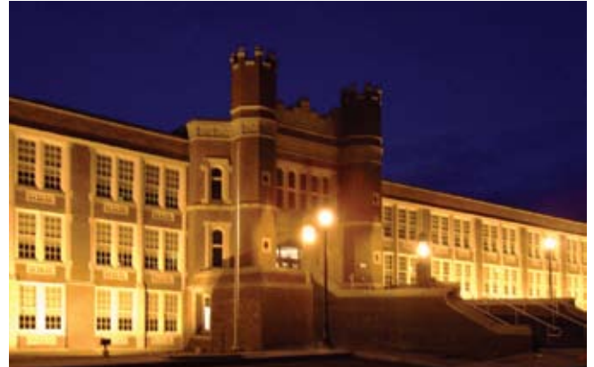
MAIN FACADE RESTORED
