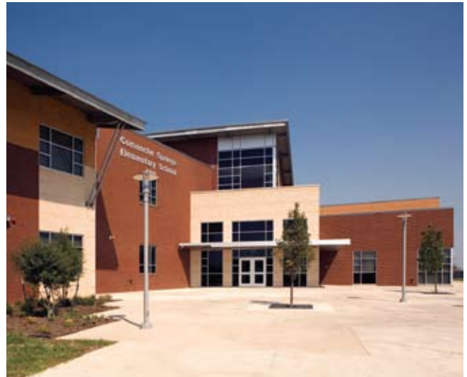
ELEMENTARY SCHOOL MAIN ENTRANCE
