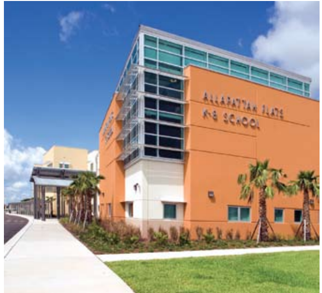
ADMINISTRATION/MEDIA BUILDING—MAIN ENTRANCE
