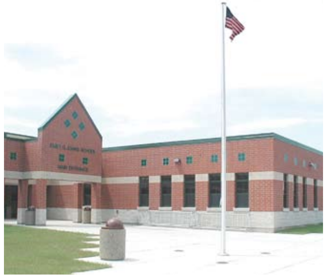
MAIN ENTRANCE EXTERIOR
