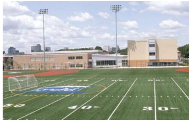
VIEW FROM BLEACHER BUILDING
