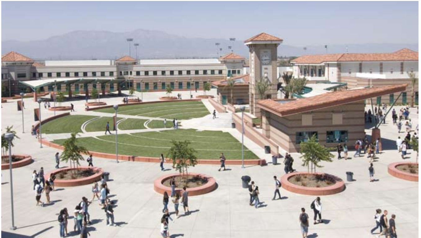
CENTRAL COURTYARD AMPHITHEATER
