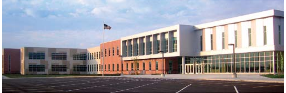
VIEW OF SOUTHWEST ENTRY PLAZA
