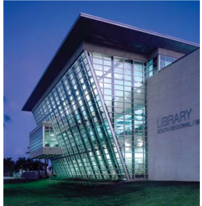
EXTERIOR NORTH ELEVATION
