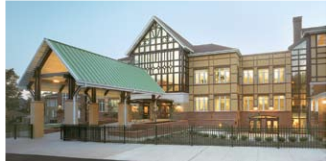
FRONT OF NEW ADDITION
