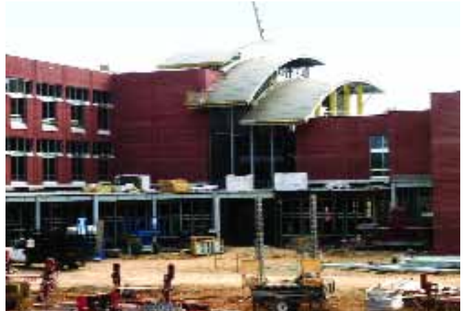
WEST ELEVATION UNDER CONSTRUCTION
