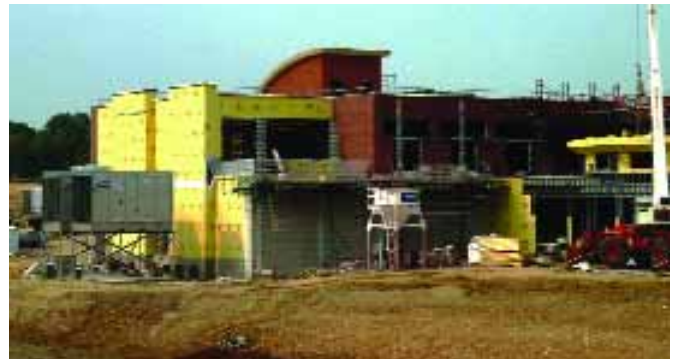
CISTERN USED FOR RAINWATER
