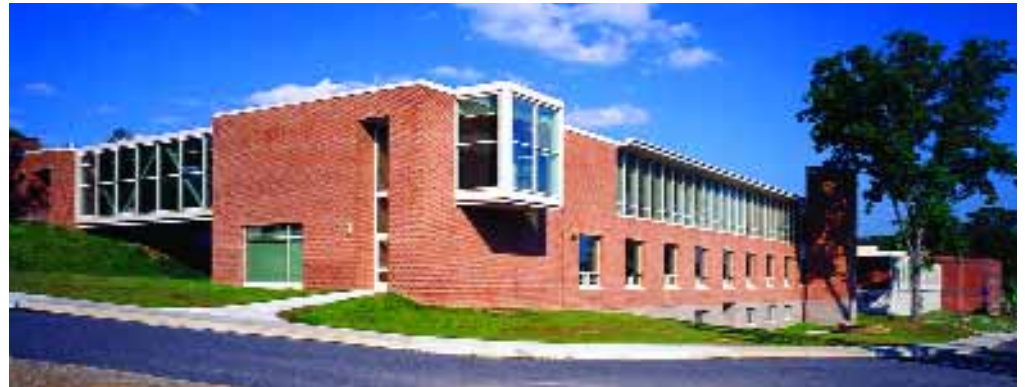
EXTERIOR OF CLASSROOM ADDITION
