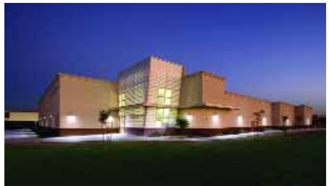
TECHNOLOGY AND INDUSTRIAL BUILDING
