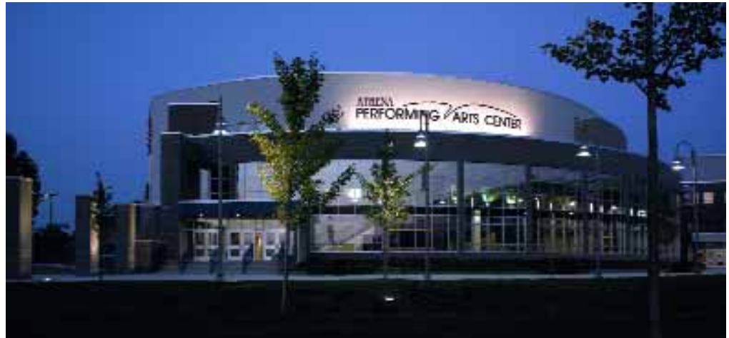
EXTERIOR ENTRANCE AT DUSK
