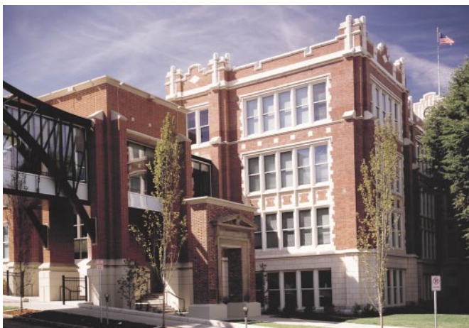
EXISTING BUILDING WITH BRIDGE CONNECTION
